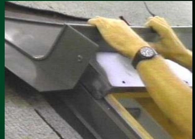
If decide to make own flashings, use lead, it's easier to work with than copper or aluminum. With little effort, bend and solder lead and solder the joints between flashings for a long lasting, watertight seal. Make paper patterns of the flashings to fit the curb; form the pieces, and then solder the joints in the saddle and apron flashings.
