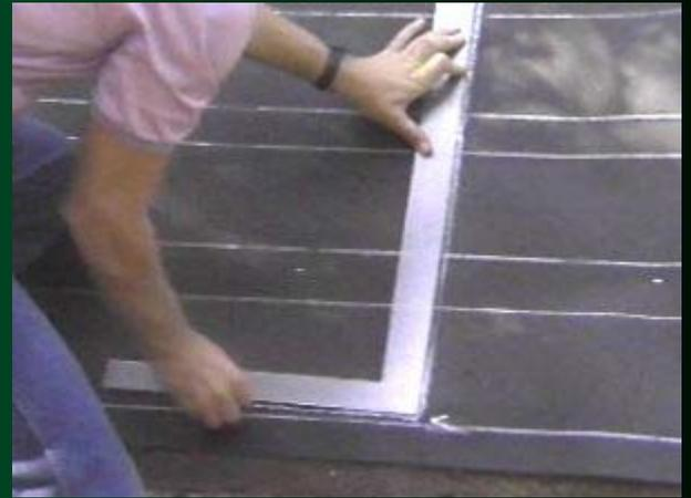
Before begin cutting through the roof, we'll have to build a curb, or box frame, for our skylight if it's the curb-mounted type. we may find it convenient to assemble the curb on the roof. If our skylight boasts an integral curb, or is self-flashing and sits directly on the sheathing, we can avoid this step.
