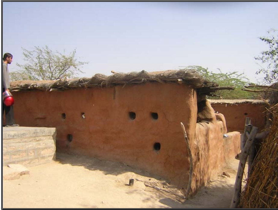
Wall construction with jalis
