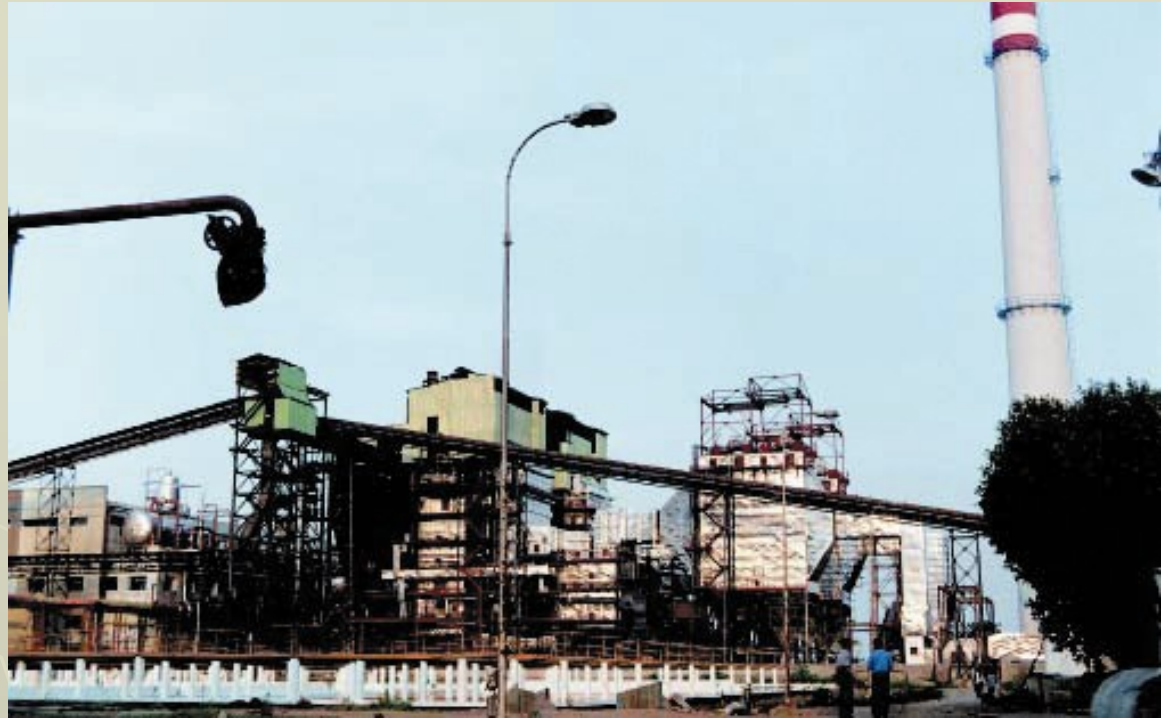
Biomass power plant in Tamil Nadu
